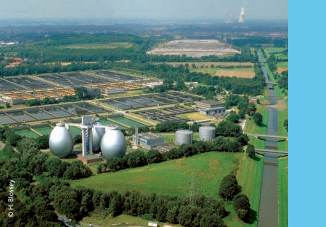
Emscher wastewater treatment plant
